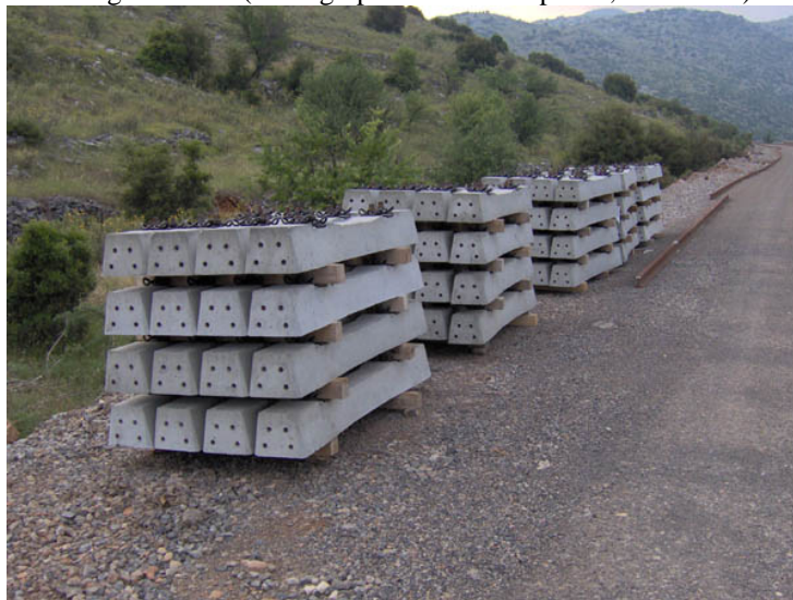
The concrete sleepers are ready to be laid just outside Kalogeriko station. Every few metres there are stockpiles like this. (Photograph: Andreas Kapaklis, June 2005)
